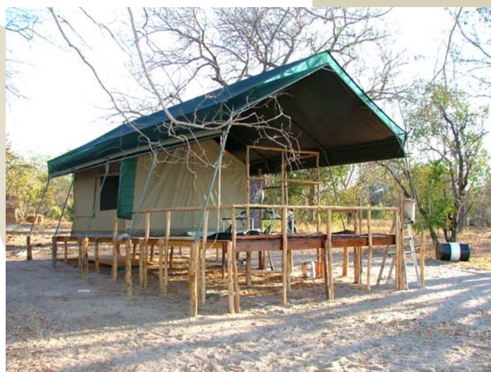
AWF is working to restore Banhine National Park in Mozambique. Construction of an International Research Center is almost complete.
